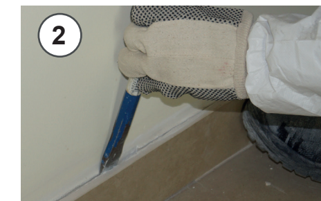
1-2-3 - Prepare the wall by removing any lamps and skirting boards, then use some cardboard to protect the floor
