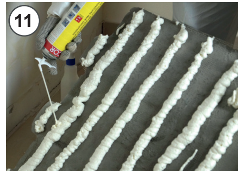
11 - Applicare la schiuma poliuretanic distanziando le strisce di circa 10 cm 11 - Application of polyurethane foam spacing the strips of about 10 cm
